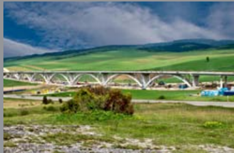
D1 Highway Bridge, Slovakia
