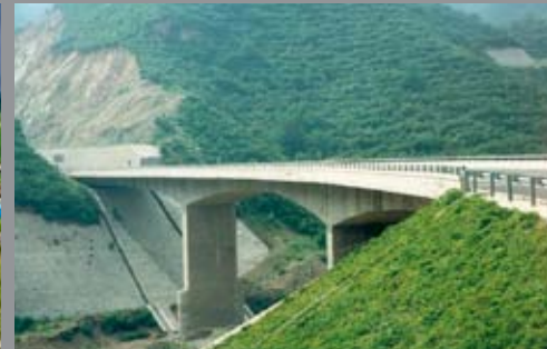
Badaling Expressway Overpass, China
