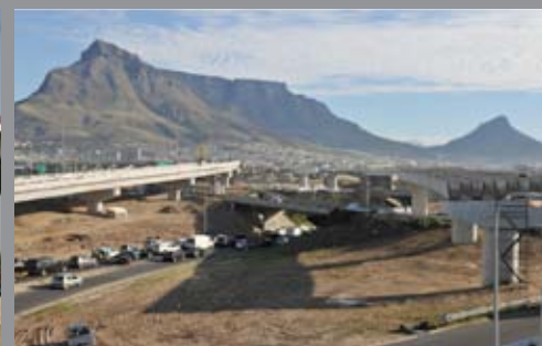
Koeberg Interchange, South Africa
