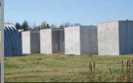
Nuclear Waste Storage Bunkers, Canada
