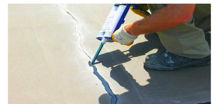
SealBoss® QuickFix Crack Repair
