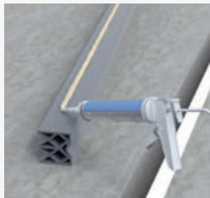
On side of the KP profile is coated with a bead of neoprene mastic.
